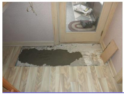
Radiant floor heat sprung a leak under the concrete slab. Fortunately, I had some experience jackhammering this slab once before.
