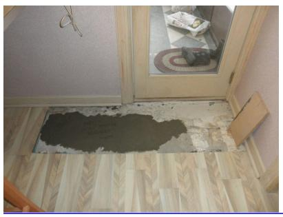
Radiant floor heat sprung a leak under the concrete slab. Fortunately, I had some experience jackhammering this slab once before.
